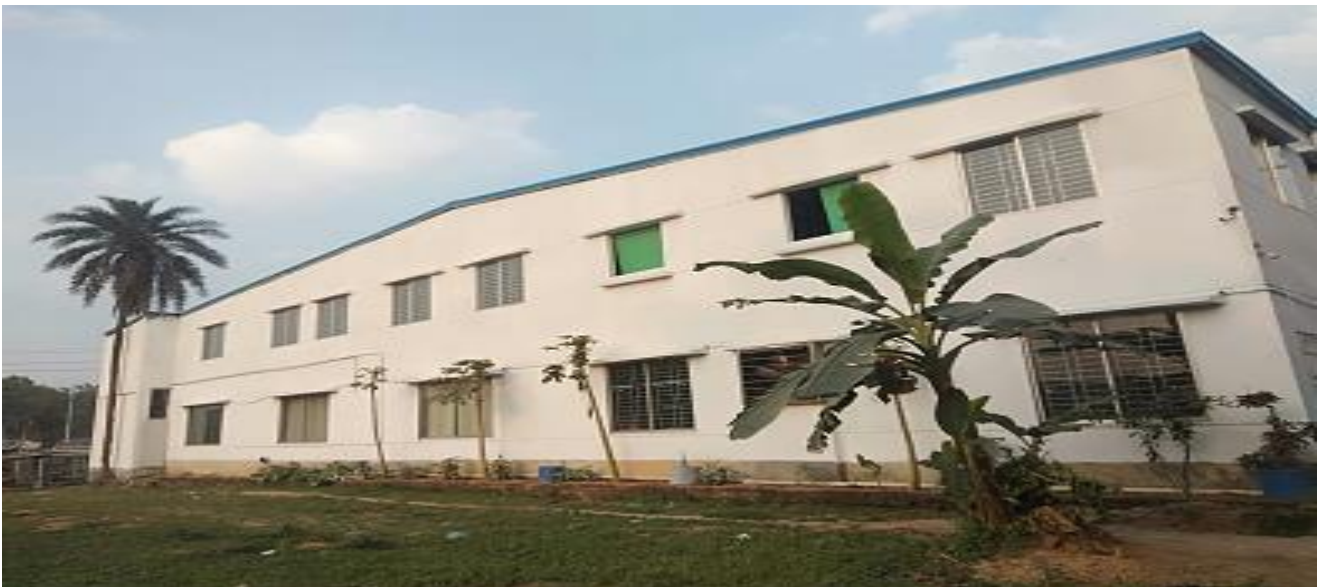
A view of west side of the factory building, picture has been taken in the year 2025
